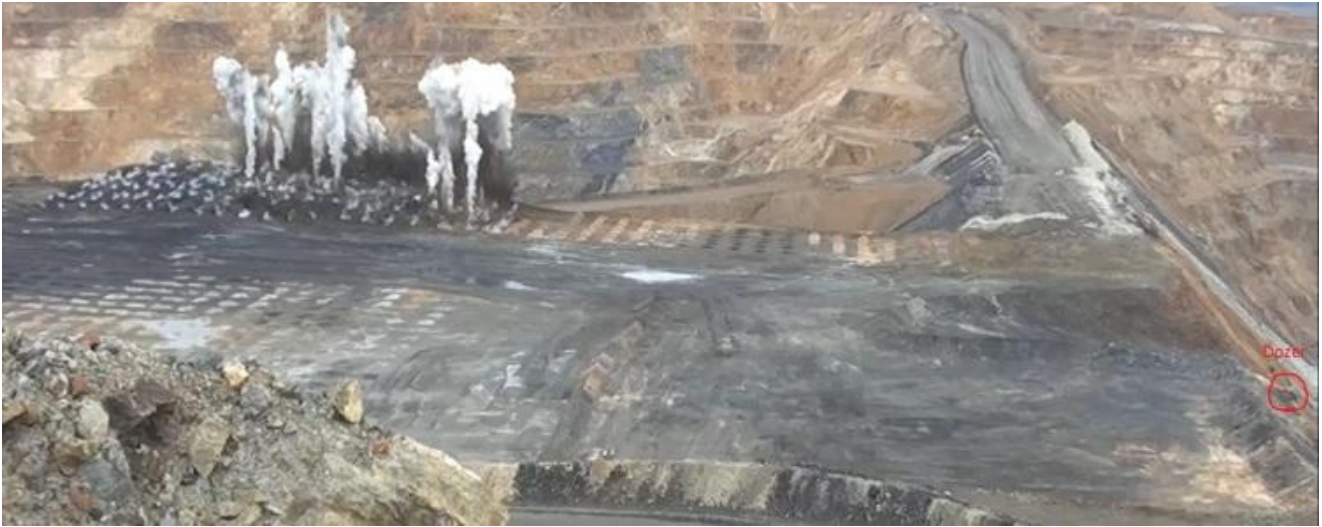
Figure 5. Second Dozer Shot
