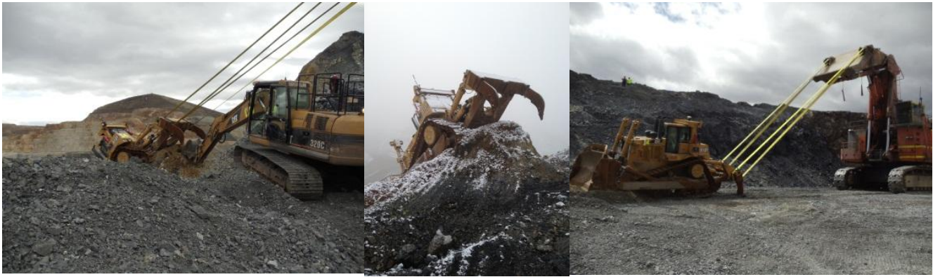
Figure 13. Dozer after Final Excavation
