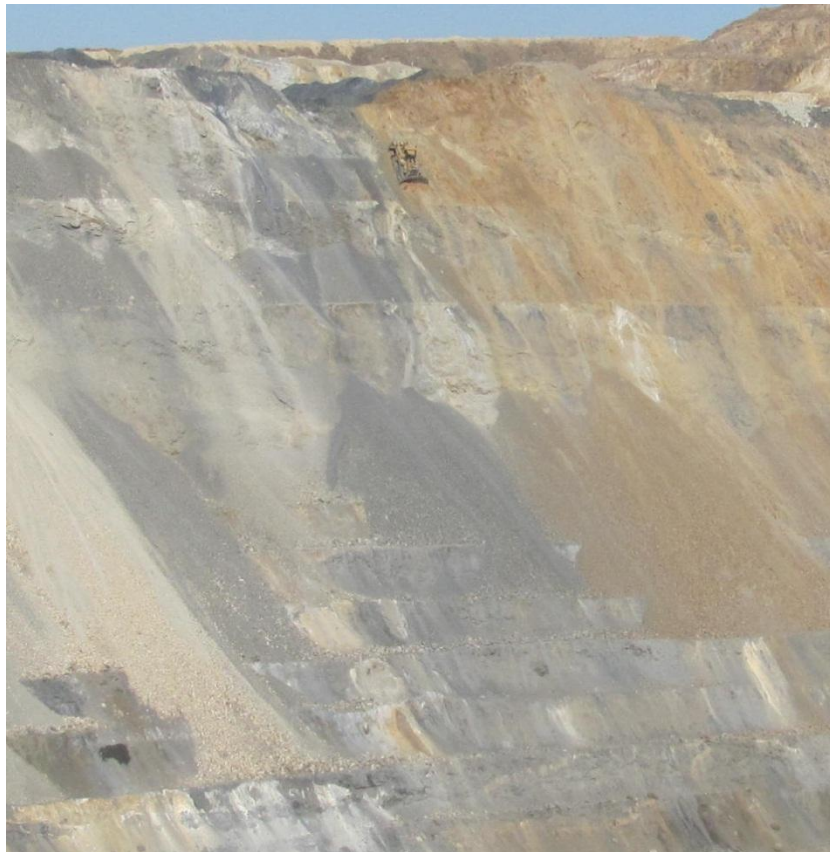
Figure 1. Day After the Dozer Drove off the Highwall
